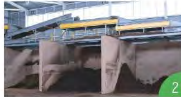
The feed stock is moved to the screening (fraction dividing) line
