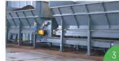
Storage tanks for raw materials of various fractions
